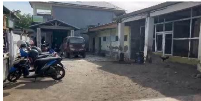
Figure 7. Actual condition of the parking area
