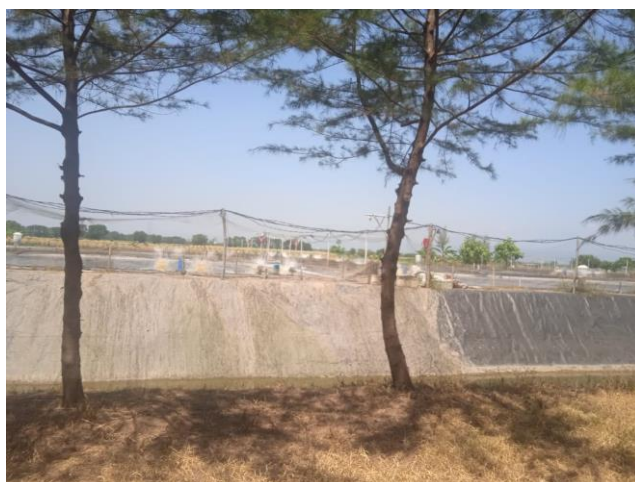
Figure 2. The Shrimp Farms at Pantai Indah Kemangi
